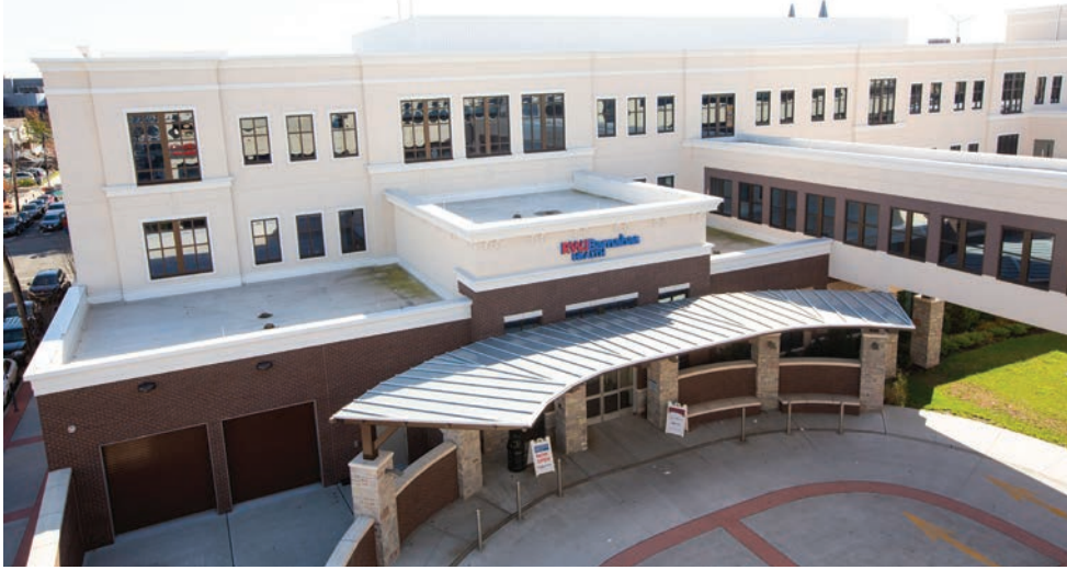
At left, the expanded RWJBarnabas Health at Bayonne building
